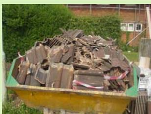
In the majority of cases we are re-using the existing roof tiles and therefore not producing significant volumes of tile rubble, however in a few instances where we do remove the tiles they are placed into a separate skip specifically for waste rubble / mortar, which is then removed from the site by Green Skips and crushed to make hardcore.
